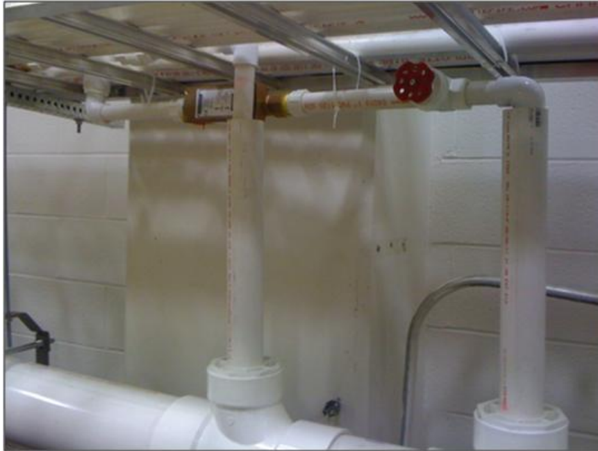
Figure 5: Discharge node configuration into the return line
