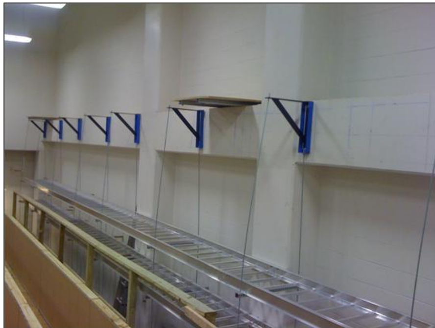
Figure 3: Pipe support structure with tank platforms
